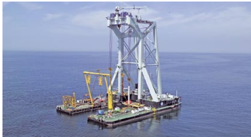
Figure A4-2: The Svanen heavy lift vessel installing foundation at OWEZ.
