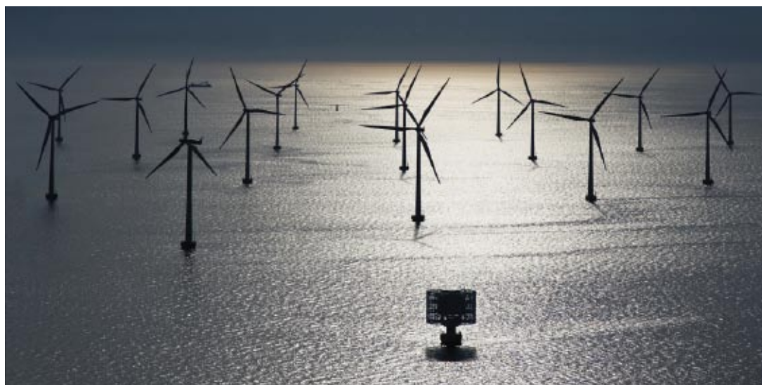
Figure A6-2: Aerial View of Lillgrund offshore wind farm. (Copyright: Siemens press picture Power)
